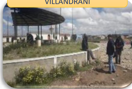
CONS PLAZA PRINCIPAL VILLANDRANI
